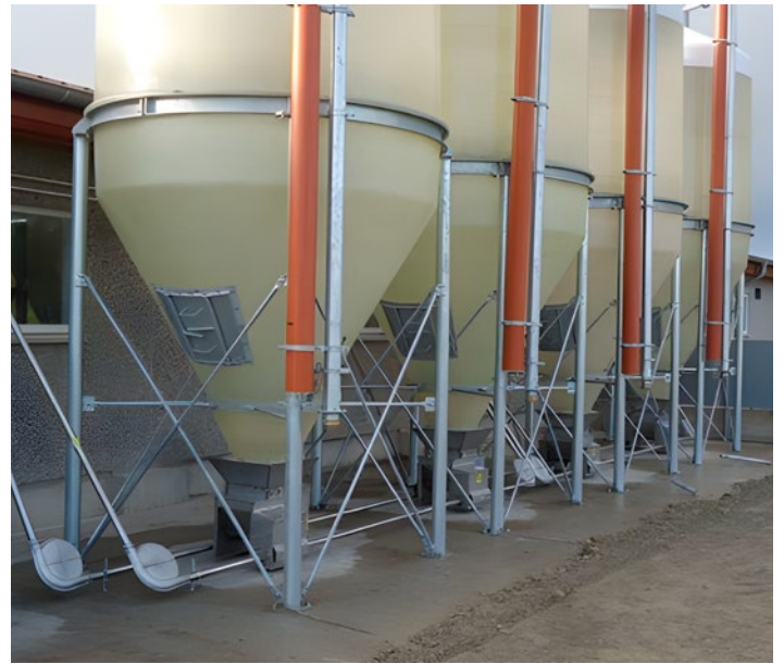
Hoppers installed on outdoor silos.
